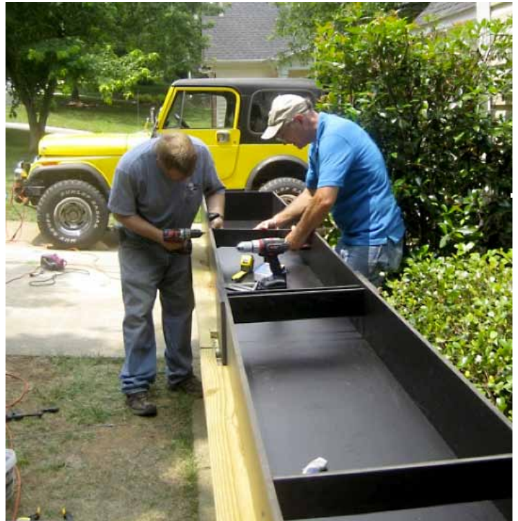
Assembling the sluice
